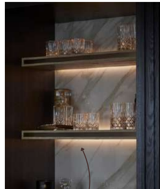
Concealed Lighting within Joinery
