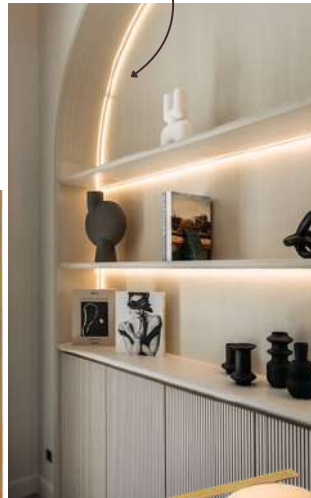
Concealed Lighting within Joinery
